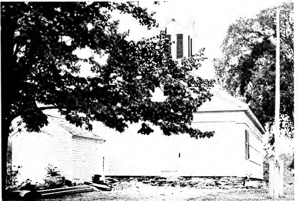
THE POMFRET LANDING SCHOOL HOUSE
